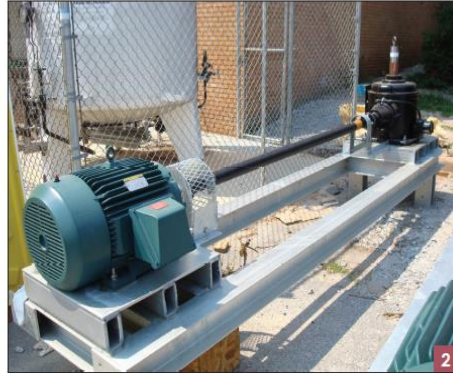
Typical fan drive arrangement.
