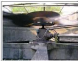
Existing Design Gearbox with Drive Shaft
