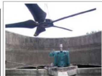
Fan Mounts Directly To Motor Shaft
